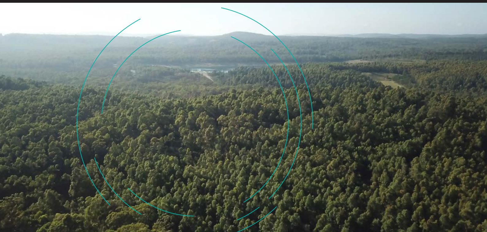
Rehabilitation of the former Westside open cut mine at the Macquarie Coal complex.
