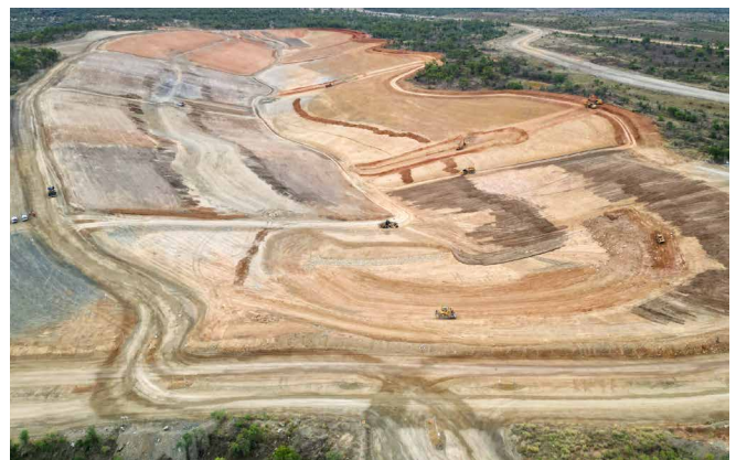
Ramp 9, showing progressive rehabilitation works – August 2024.
