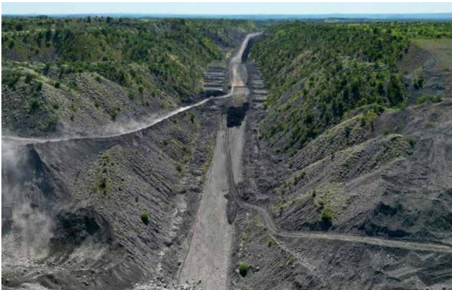
Ramp 10 looking up the ramp – February 2023.
