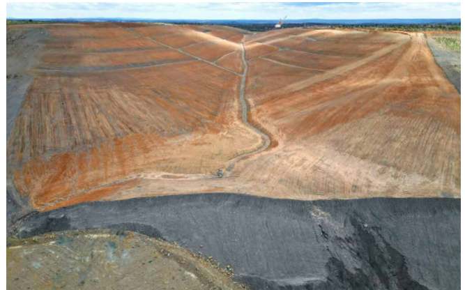
Ramp 10, showing progressive rehabilitation works – August 2024.
