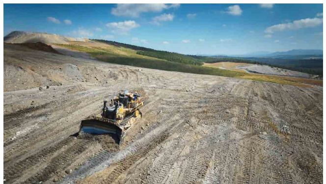
Rehabilitation work being conducted at Ravensworth Open Cut.
