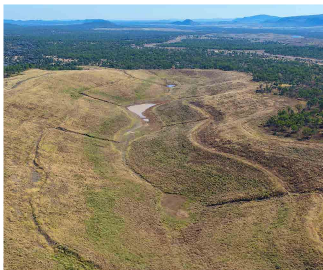
Ramp 9, showing progressive rehabilitation works – August 2025.
