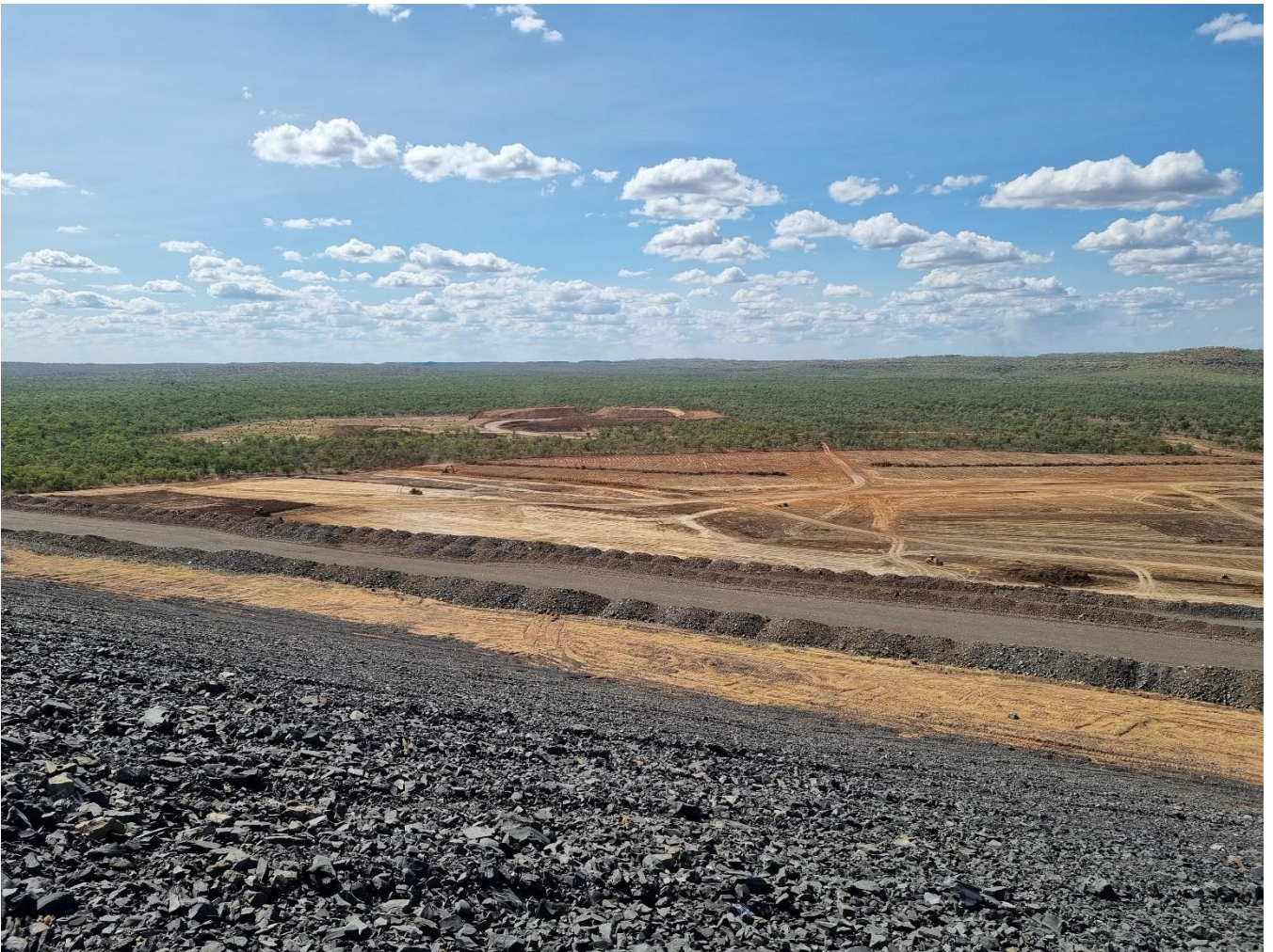
Photograph 7 - NOEF expansion civil works
