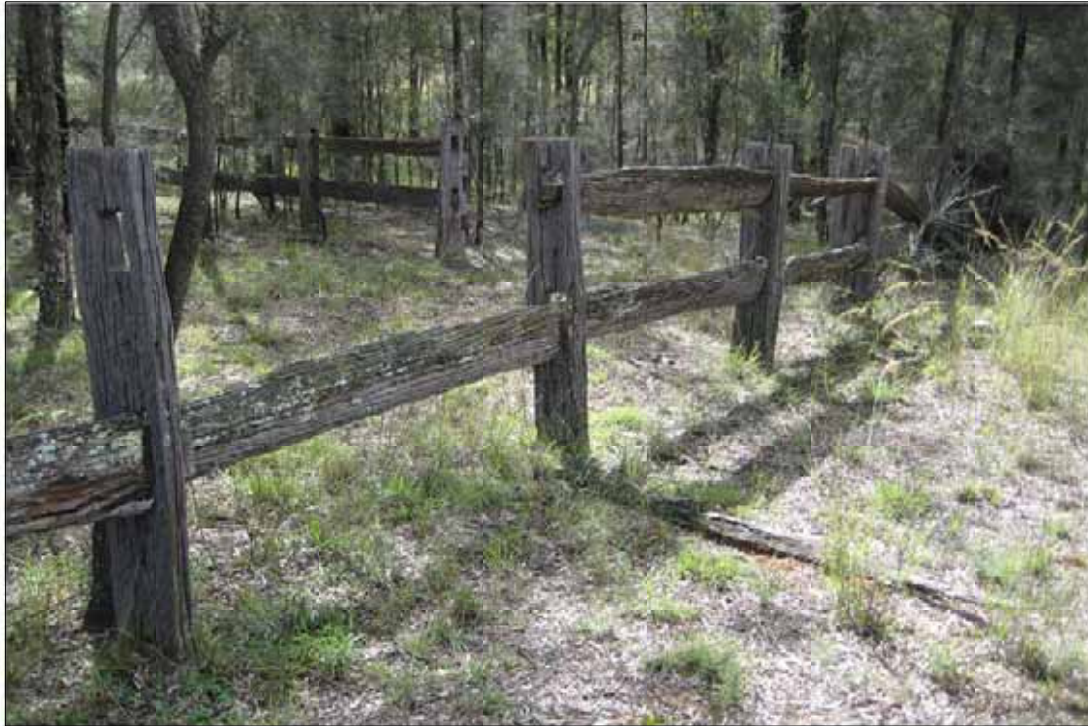
PLATE 4.7 View of site/item HH5 - mortise and tenon post and two-rail fence enclosure adjacent to dam
