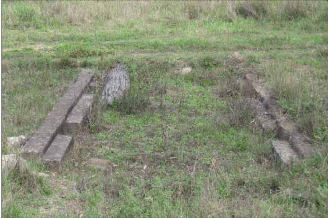
PLATE 4.13 View of site HH13 - concrete foundations alongside vehicle track
