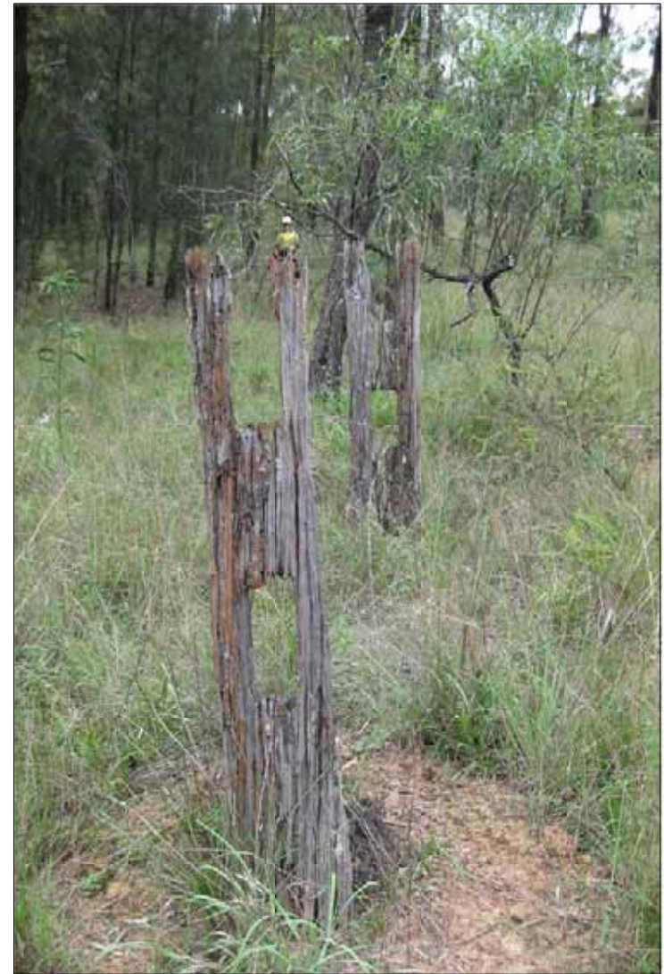
PLATE 4.8 View of site HH6 mortise and tenon post fence line
