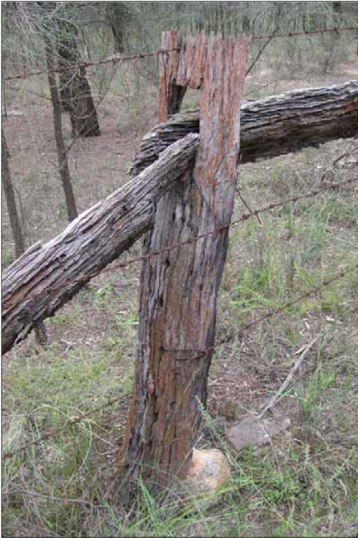
PLATE 4.19 View of site/item HH17 - detail showing wire hooked through drill hole/through mortise joint to attach wire fencing
