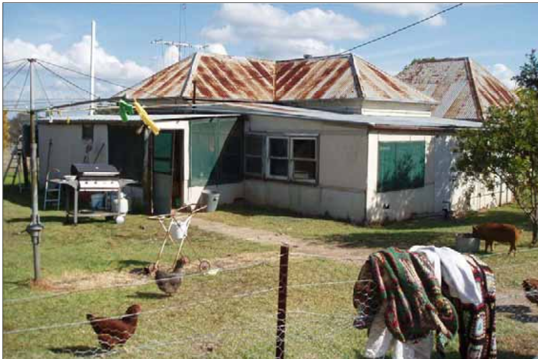
PLATE 4.14 View of site/item PK 243 (Apple Tree Flat farm complex). Original mid to late nineteenth century constructed cottage shown to rear with steeper pitched roof
