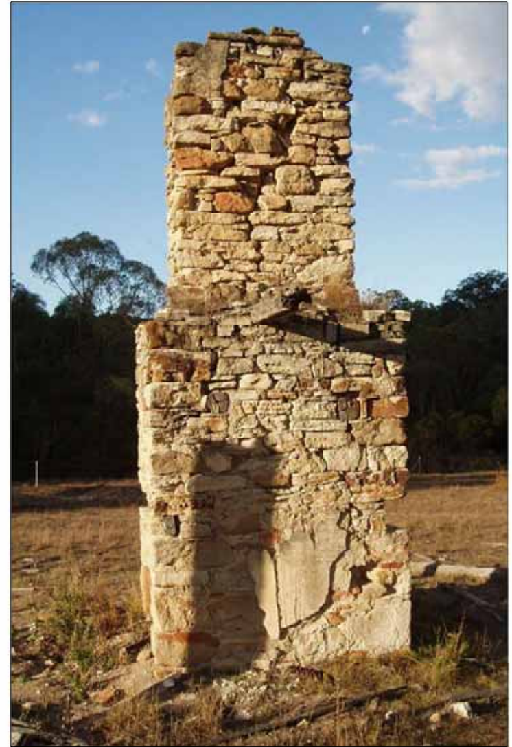
PLATE 4.4 Detail of remnant stone chimney of former hotel of Old Ulan Village
