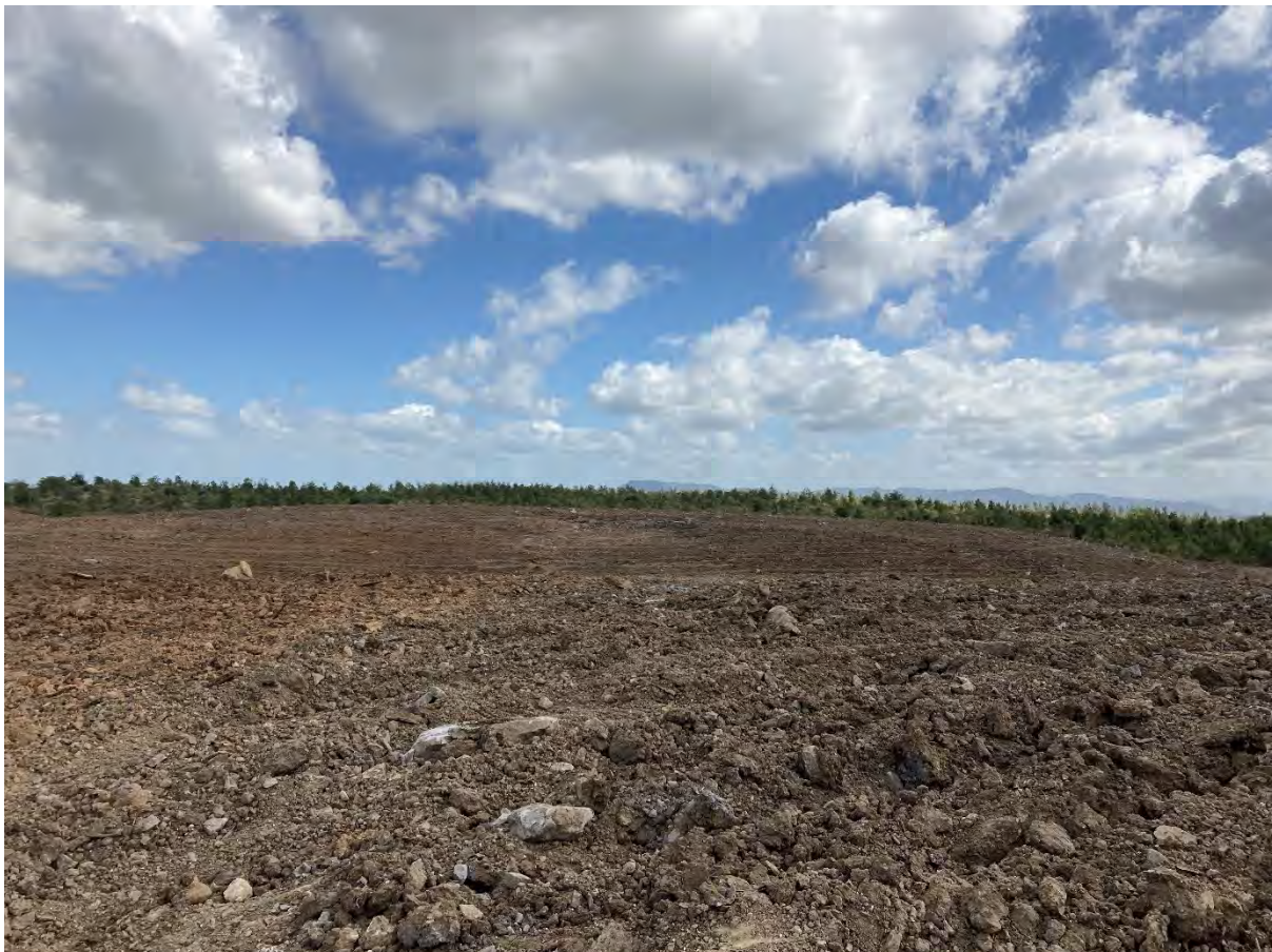
Photo 6 – Rehabilitation Progress 2022. Western Emplacement Area
