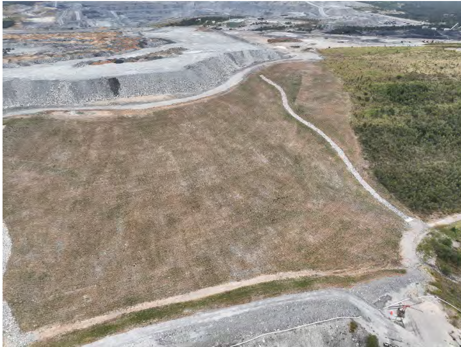
Photo 1 – Rehabilitation Progress 2022. Eastern Rehabilitation Area
