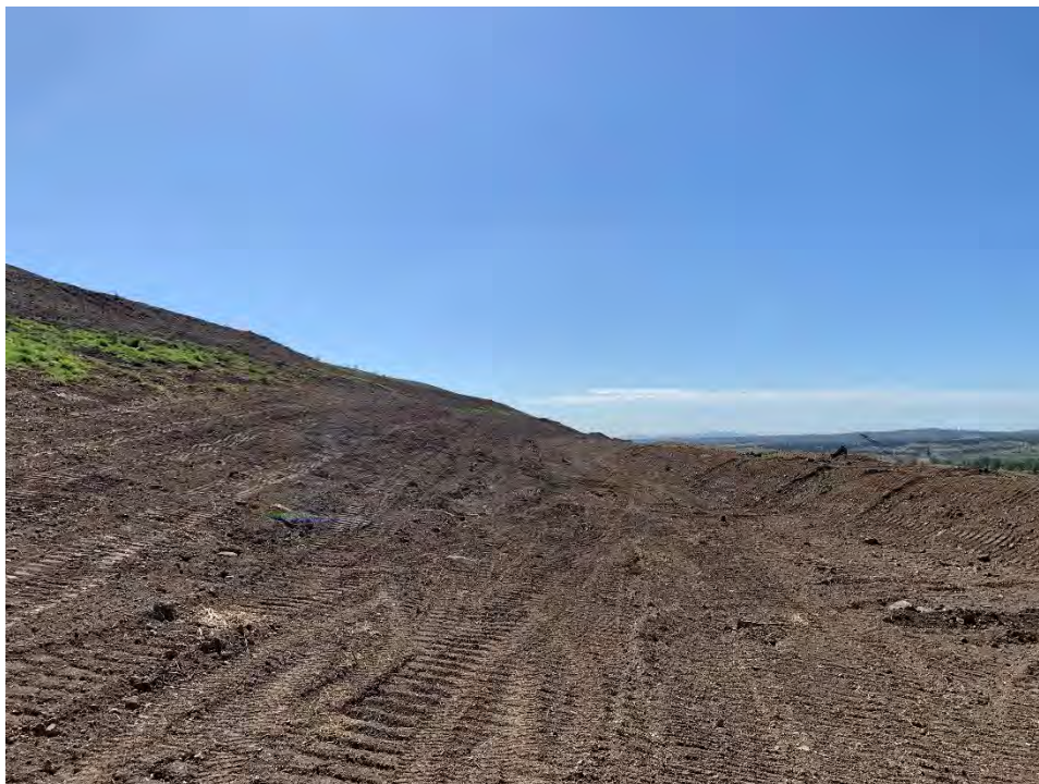
Photo 4 – Rehabilitation Progress 2022. Narama Rehabilitation Maintenance
