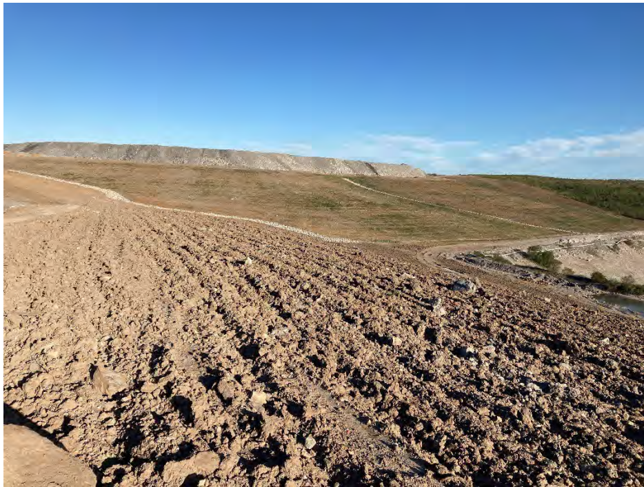
Photo 3 – Rehabilitation Progress 2022. Eastern Rehabilitation Area
