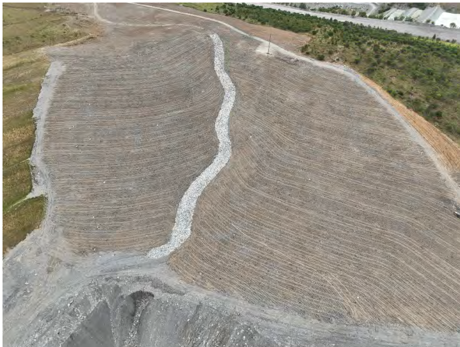
Photo 2 – Rehabilitation Progress 2022. Eastern Rehabilitation Area
