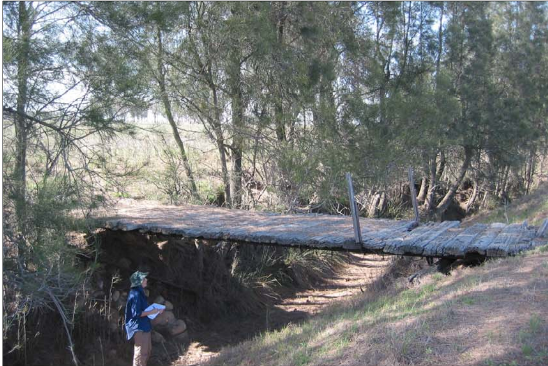
PLATE 3.1 Wooden Bridge, Swamp Creek (Item 1) MGA 318354, 6408595
