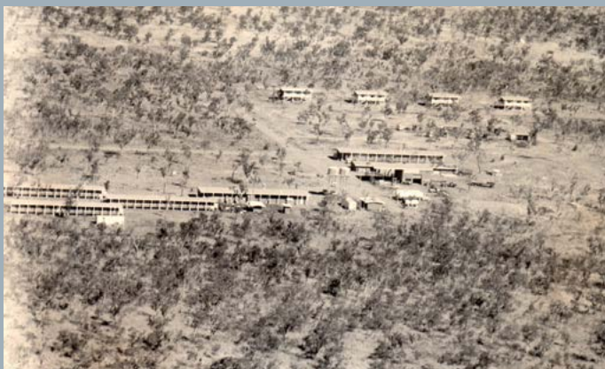
1960s The main camp, looking from the south. The main kitchen and barracks are in the left of the photo.
