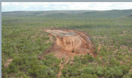
Work begins on the McArthur River channel.
