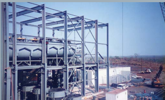
1994 The flotation building under construction.
