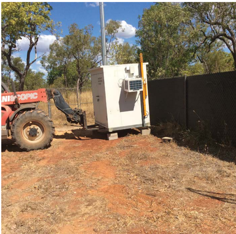
The new Air Quality Monitoring Station being installed at Borroloola
