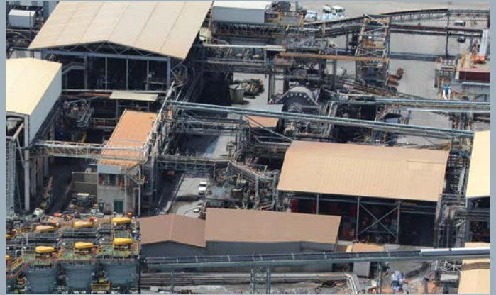
2015 The SAG mill can be seen in the centre of this photo surrounded by new mill components.
