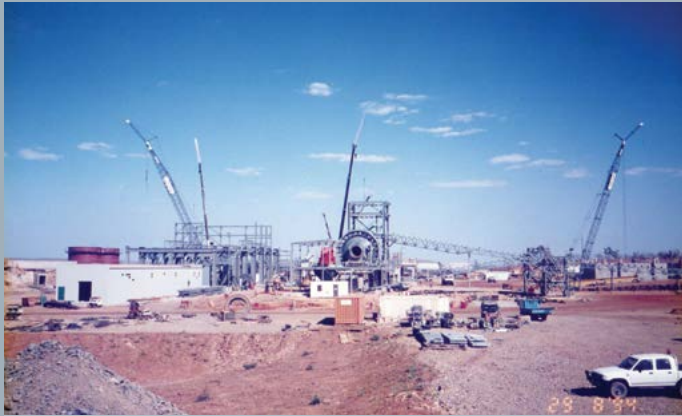
1994 The SAG mill is under construction in the centre of this photo.
