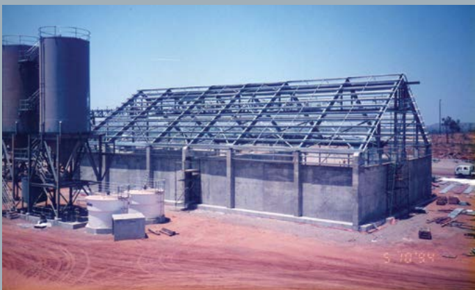
1994 The concentrate storage shed under construction with the lime silos and flocc tanks to the left.
