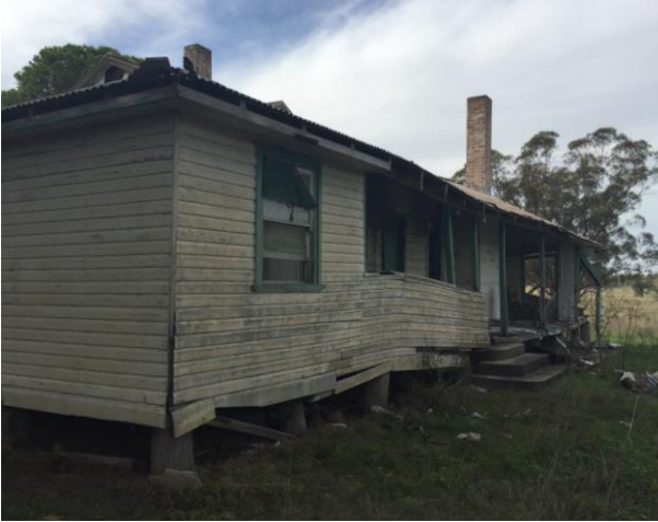
Figure 11 Front (southern) facade Hillcrest
