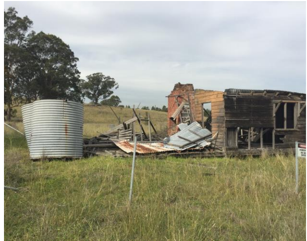
Figure 16 Rear and western facade of the cottage
