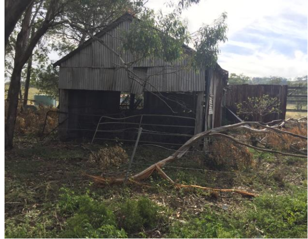
Figure 12 Garage to the north west of the main house
