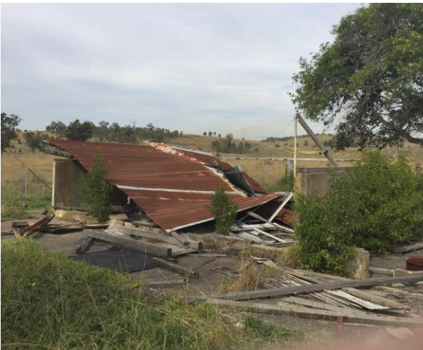
Figure 6 View of the shed to the south east
