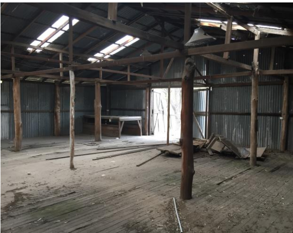
Figure 13 Interior shearing shed
