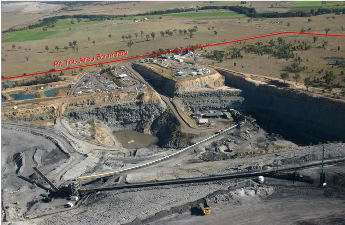
Plate 2.3: An oblique aerial view to the northwest towards the Portal Area and Pit Top Facilities. Ref: E642-F056
