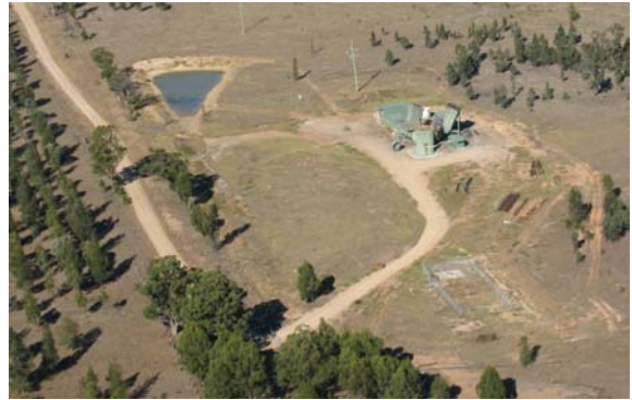
Plate D Forest Road Ventilation Shaft Area
