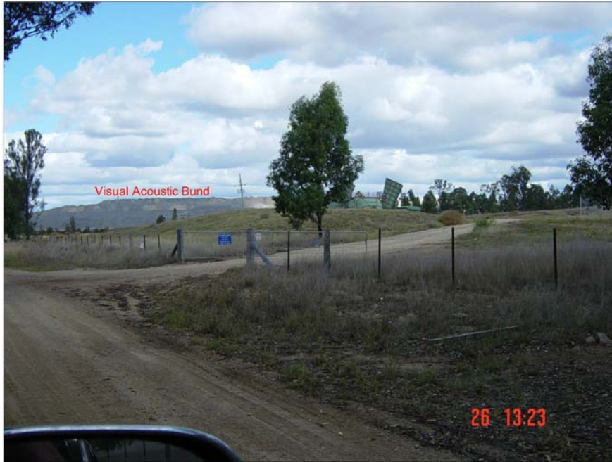
Plate 2.9: The Forest Road Ventilation Shaft Facilities looking south-southwest from Forest Road. The Ashton out-of-pit overburden emplacement lies in the background. Ref: DSC 01124.jpg
