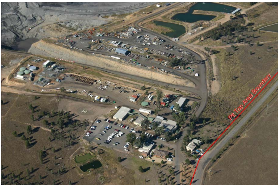
Plate 2.4: An oblique aerial view to the south across the Pit Top Facilities. Ref: E642-F129
