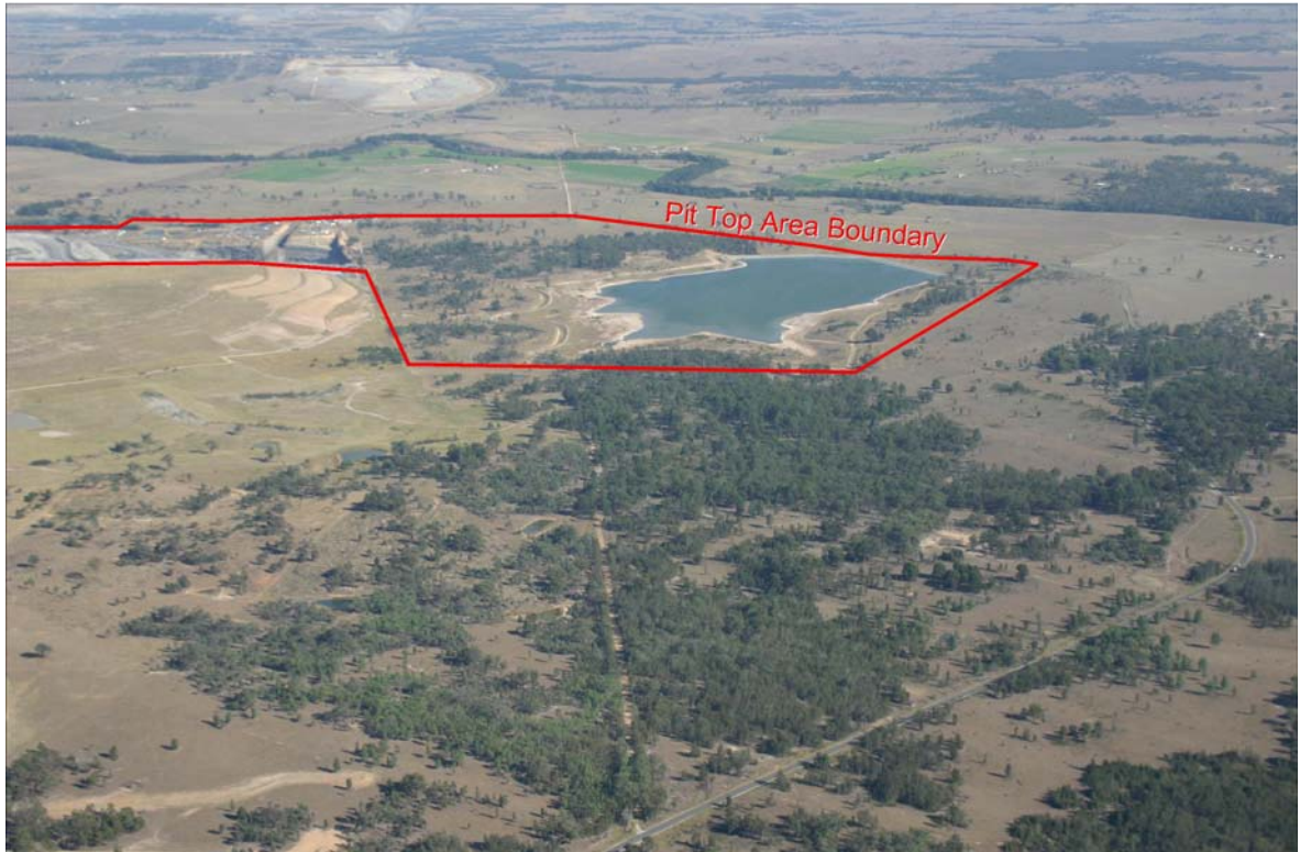
Plate 2.1: An oblique aerial view to the northwest towards Glennies Creek Colliery Pit Top Facilities (left) and Possum Skin Dam (centre) Ref: E642-F107
