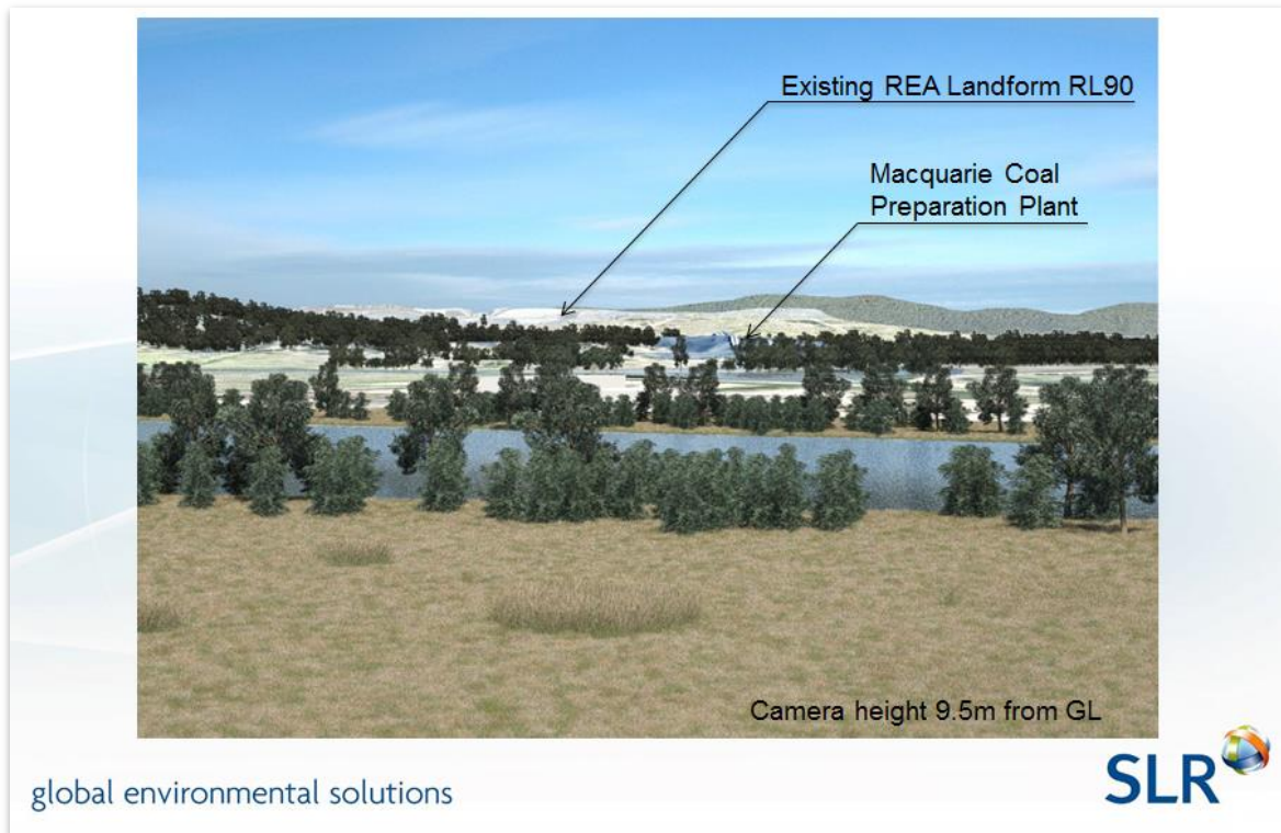
Figure 4 Existing view from TC Frith Avenue, Boolaroo (note camera height is 9.5m from ground level)
