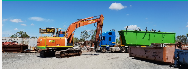
Zebra Metals undertaking site wide waste metal cleanup.
