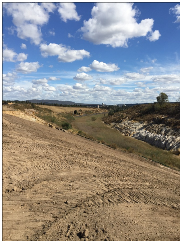
Plate 8 Goulburn River Diversion Remediation Works 1
