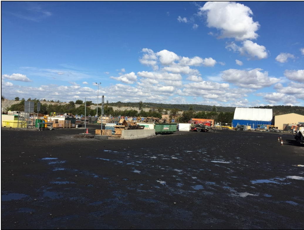
Plate 5 Hard stand area well maintained and watered
