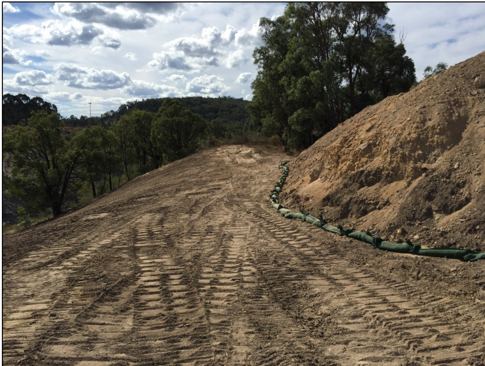
Plate 9 Goulburn River Diversion Remediation Works 2
