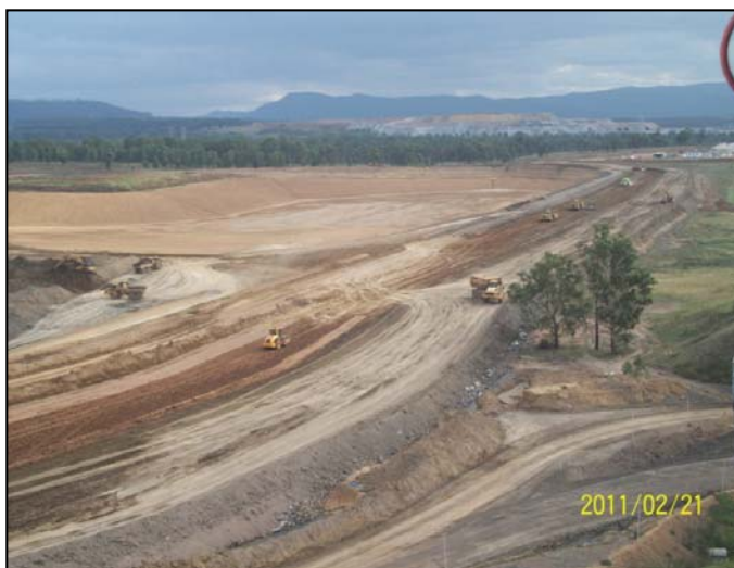
Plate 2.3 – Construction of CHPP Surge Dam
