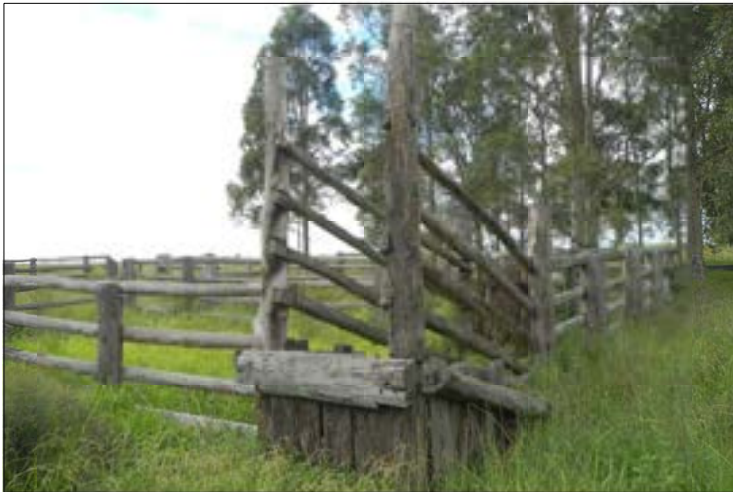
PLATE 4.19 View to south-east site MOH7 timber yards
