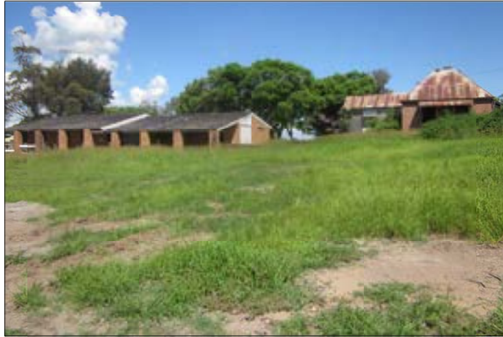
PLATE 4.5 View to south - 1880 and 1971 constructed Ravensworth Public School buildings
