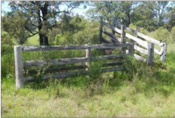
PLATE 4.25 View to north-west site MOH9 yards
