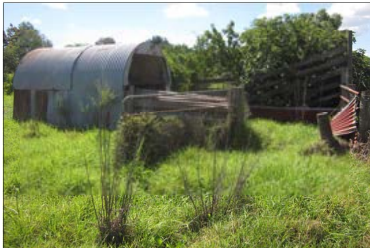
PLATE 4.11 View to north Ravensworth Village animal enclosure
