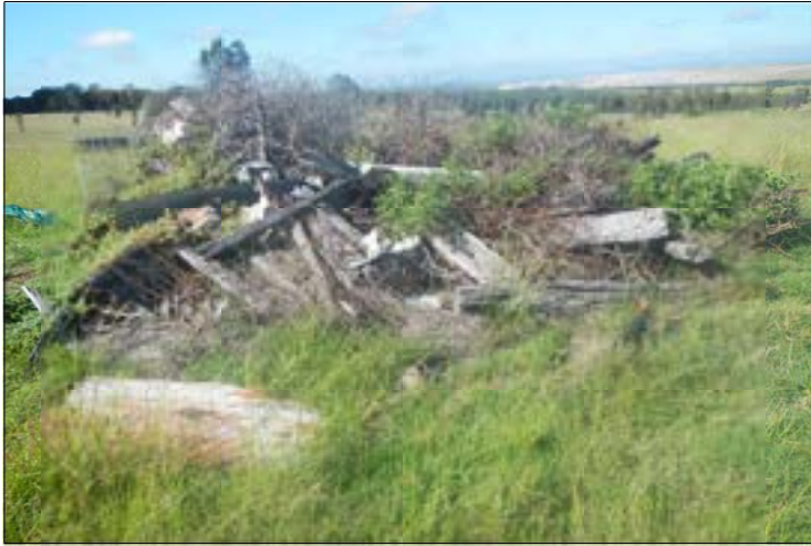
PLATE 4.17 View to west site MOH6 demolition rubble
