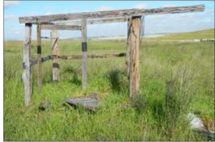
PLATE 4.18 View to west site MOH6 timber frame
