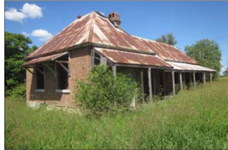
PLATE 4.6 View to south-east - 1880 constructed Ravensworth Public School building
