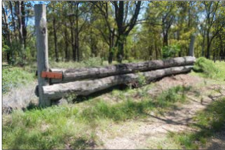
PLATE 4.29 View to north-west site MOH10 timber loading ramp
