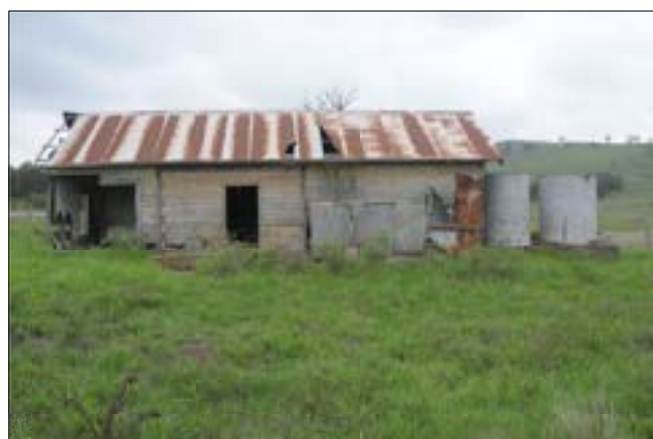
PLATE 4.3 View to north - MOH5. Photograph dated January 2010
