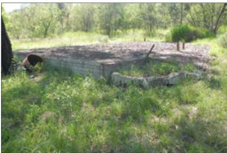
PLATE 4.28 View to north-east site MOH9 concrete slab
