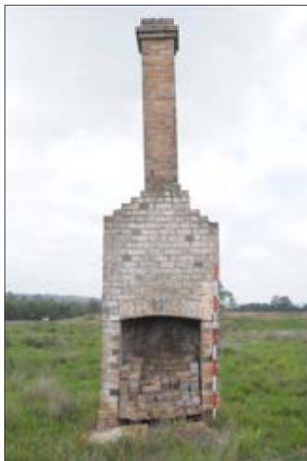
PLATE 4.1 View to south - MOH5. Photograph dated January 2010
