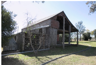
Image 20 Carriage House: shingles and battens under metal roofs.
