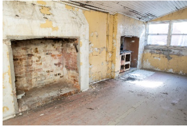
Image 14 Kitchen Wing: Interior. Recently cleaned out and swept.
