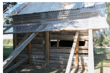
Image 09 Butcher's Hut: temporary stabilisation works and protection of structure.
