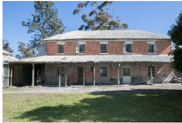
Image 17 Kitchen Wing: east elevation. Propping has been installed throughout.
