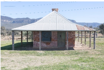
Image 22 Stud Masters': Tarpaulin removed, new roof reconstructed.
