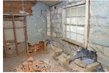
Image 15 Kitchen Wing: Interior. Walls propped, materials retained in their location.
