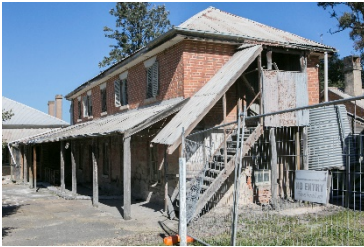
Image 16 Kitchen Wing: north east corner.
