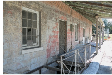
Image 18 Kitchen Wing: stairs down to the cellar. Sandbagging installed to divert water away.
