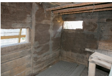
Image 10 Butcher's Hut: Interior cleaned out and self seeded plant removed.
