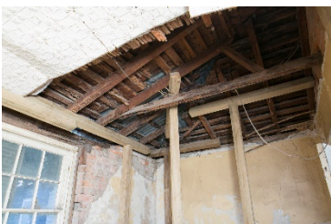
Image 07 New House: shingle roofing, pressed metal ceilings and other "layers" evident.
