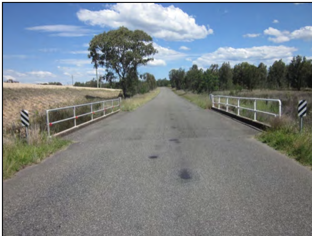
Figure 58: Looking south over the bridge at MGA 317618/63 (IMG 1652).
