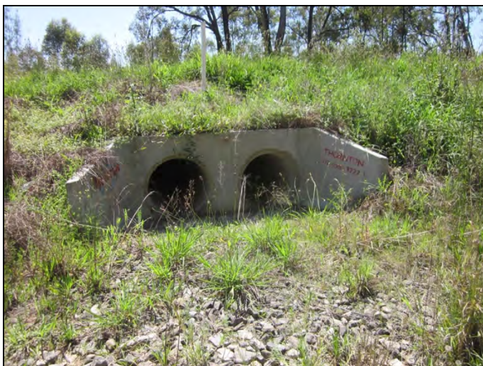
Figure 36: Two pipe concrete culvert at MGA 319232/6381074 (IMG 1464)
