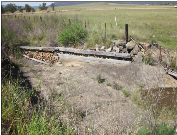
Figure 29: Bank stabilisation at the above culvert, looking west (IMG 1431).
