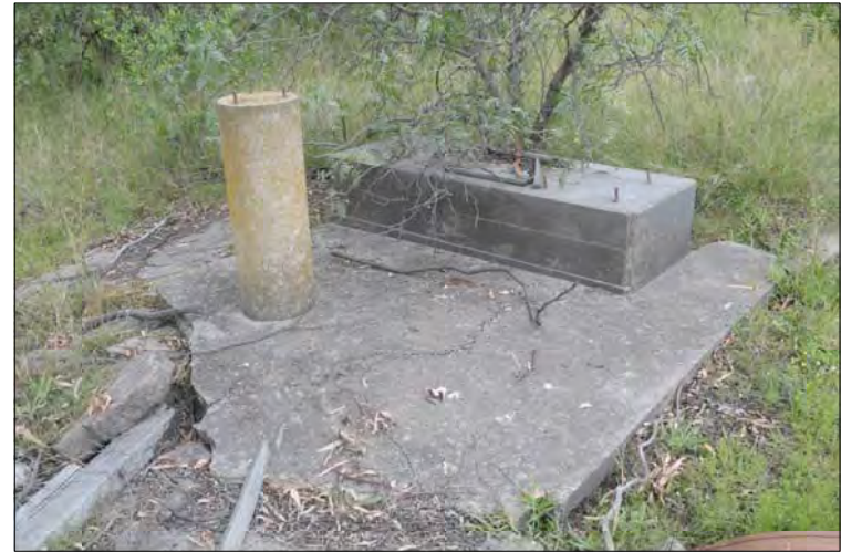
PLATE 4.18 PS6 concrete slab, view to South-East
