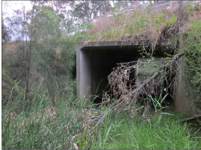
PLATE 4.61 Bridge culvert over Nine Mile Creek, view to West
