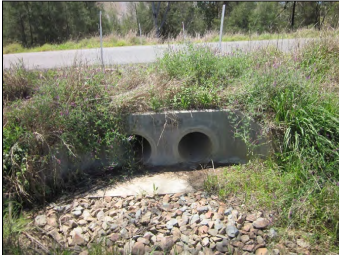
Figure 42: Two drain culvert, looking east at MGA 318555/6382728 IMG 1526).
