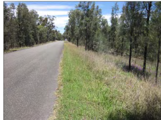
PLATE 4.48 Area of embankment within area to be realigned, view to South
