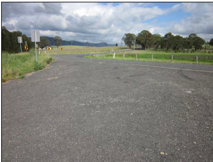
Figure 19: Intersection of the original line of road with the current Charlton Road (IMG 1208).
