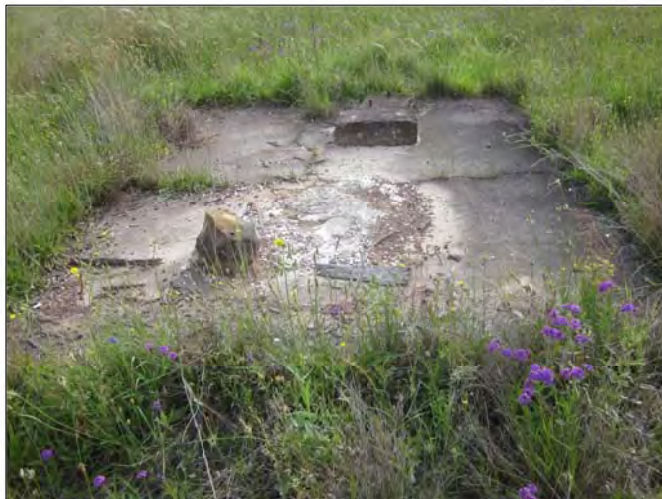
PLATE 4.3 BH11 concrete slab, view to North-East
