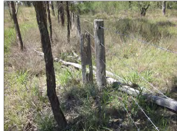
PLATE 4.64 BH2 fence posts along Charlton Road, view to South
