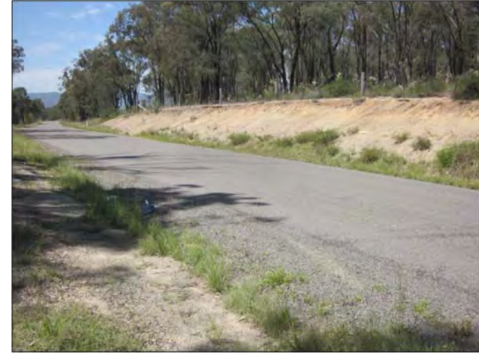
PLATE 4.50 Area of cutting (to South of) area to be realigned, view to South
