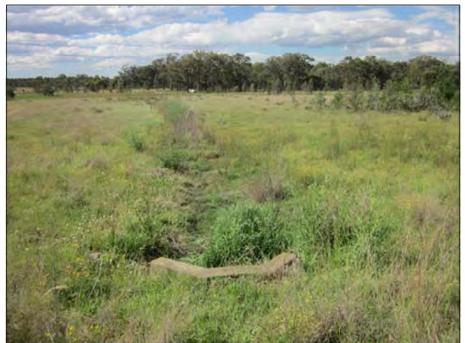
PLATE 4.56 Culvert association with former Broke Airstrip, view to North towards forested area
