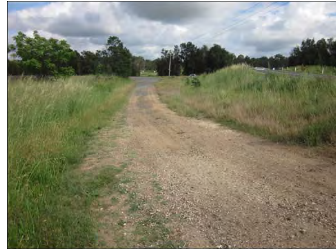
PLATE 4.38 Section of abandoned Great North Road at Monkey Place Creek, view to North-West
