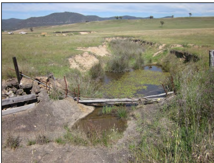
Figure 30: Creek channel at the above culvert, looking to the west (IMG 1432).
