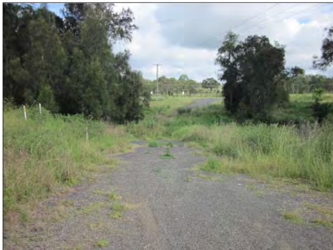
PLATE 4.39 Section of abandoned Great North Road crossing Monkey Place Creek, view to North-West
