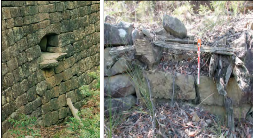
Figure 72: Stone culvert in retaining wall, Devine's Hill.
