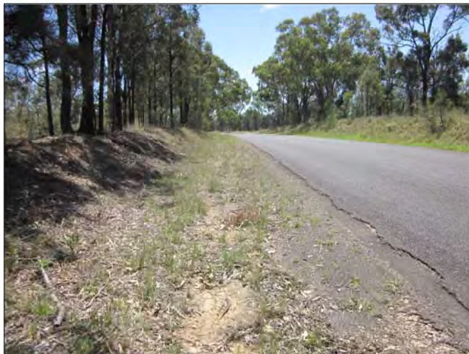
PLATE 4.47 Area of cutting within area to be realigned, view to North
