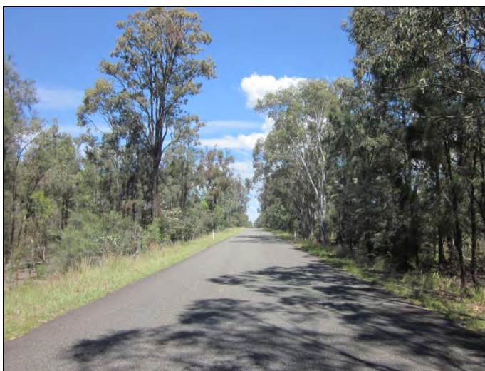
Figure 56: Looking south from the end of the proposed realignment at MGA 317828/6384882 (IMG 1680).
