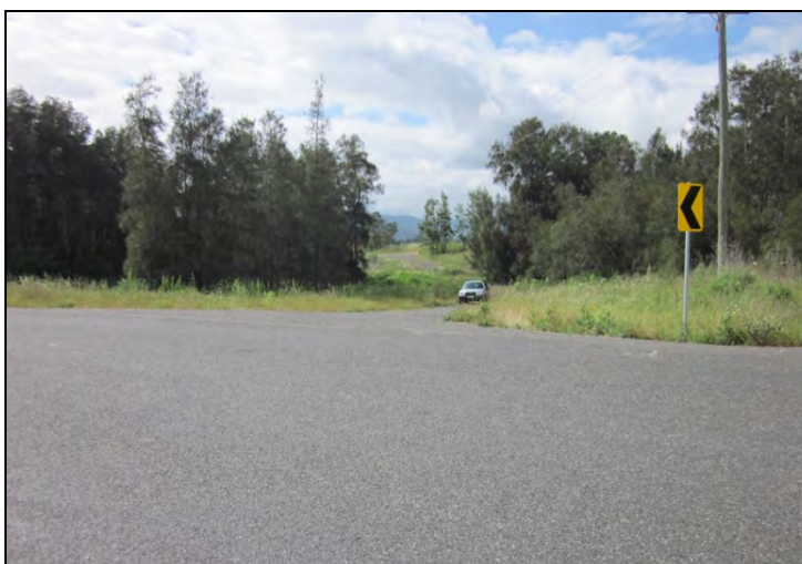
Figure 20: Intersection of the original line of road with the current Charlton Road, looking south east (IMG 1223).
