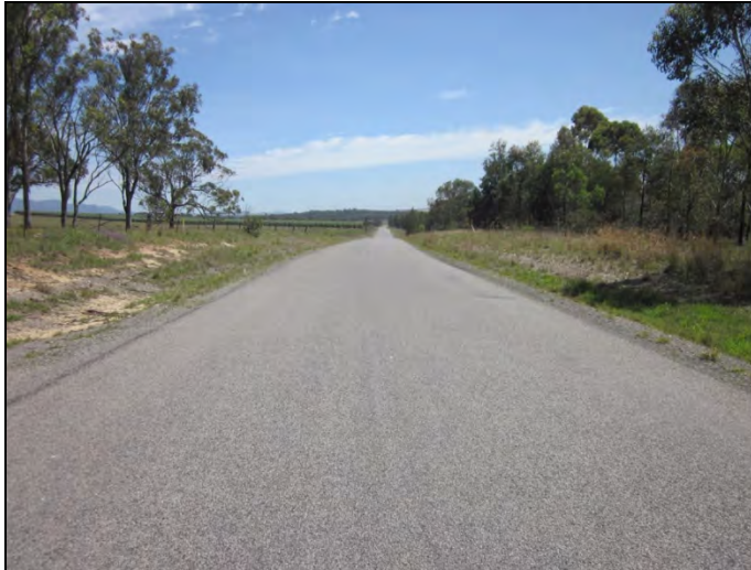
Figure 39: Looking north from the above culvert (IMG 1502).
