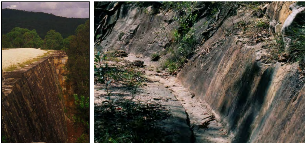
Figure 70: Retaining wall and buttress, Devine's Hill.
