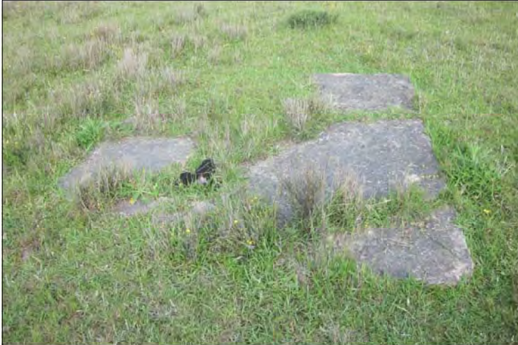
PLATE 4.25 PS10 concrete slab, view to West
