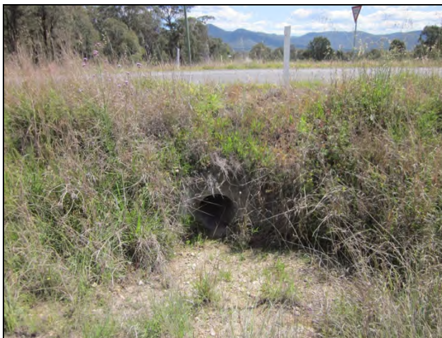
Figure 68: Culvert at intersection with the Putty Road, looking east (IMG 1688).
