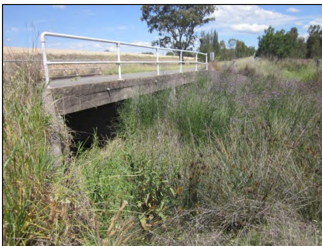
Figure 59: Detail of the culvert beneath the above bridge, looking south east (IMG 1653).
