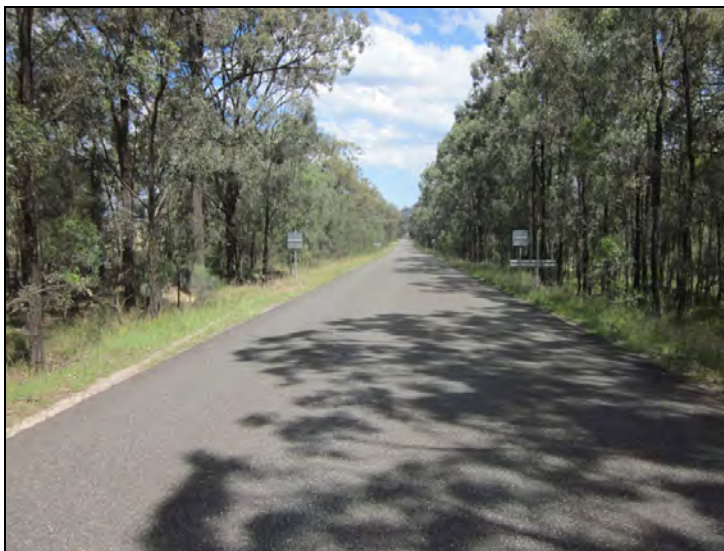
Figure 64: View south along the road from the above culvert (IMG 1680).
