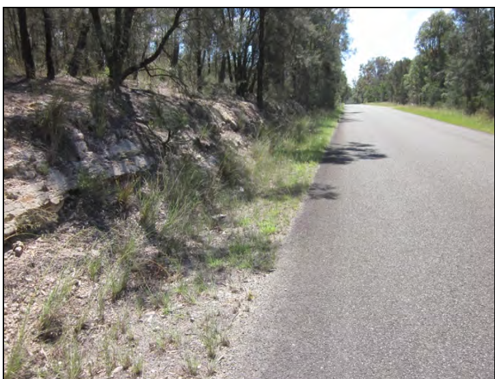
Figure 53: Cut on the western side of the road, looking north at MGA 317984/6384572 (IMG 1626).
