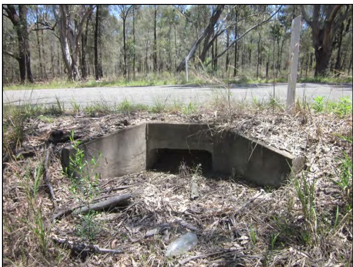
Figure 47: Modern concrete culvert on the eastern side of the road at MGA 318170/6384064 (IMG 1591).
