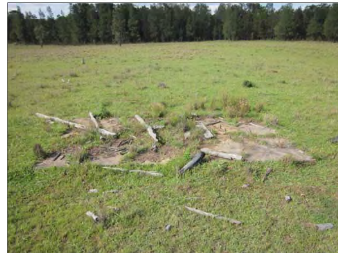
PLATE 4.24 PS10 concrete slab, view to North
