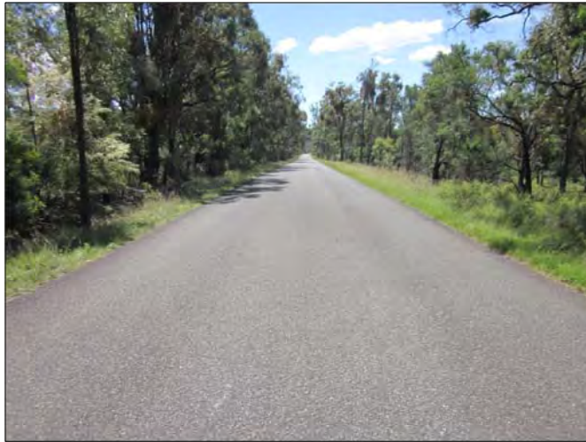
PLATE 4.45 Typical straight section of road within area to be realigned, view to North
