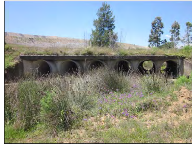
PLATE 4.42 Six-pipe culvert under Charlton Road, within realignment area, view to East
