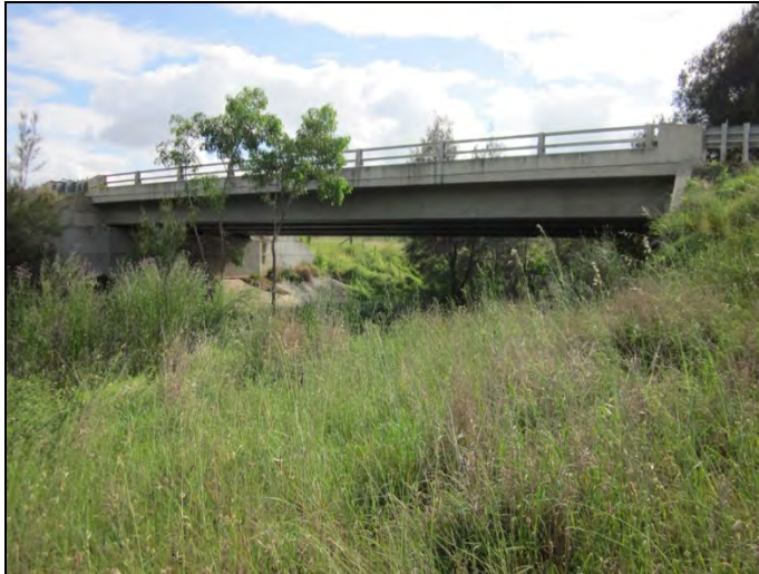
Figure 15: The current line of road where it crosses Monkey Place Creek (IMG 1193).
