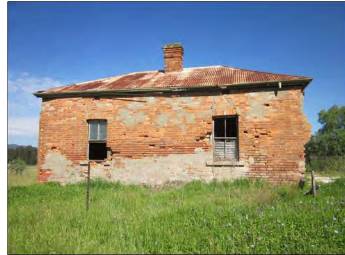
PLATE 4.66 BH7 McNamara's Dairy Cottage, view to West
