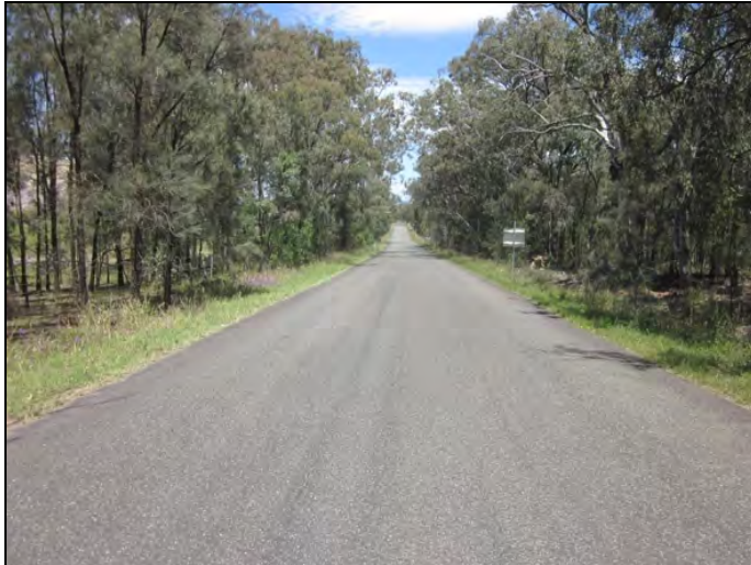
Figure 48: View along the road to the north from MGA 318170/6384064 (IMG 1594).
