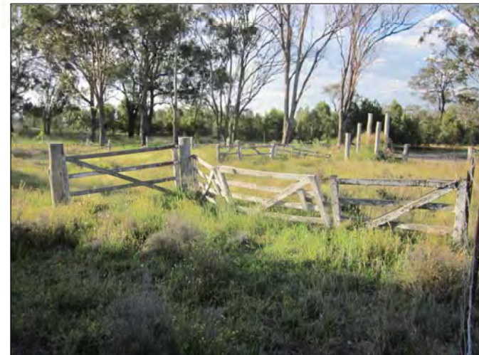
PLATE 4.32 PS16 timber yards, view to West
