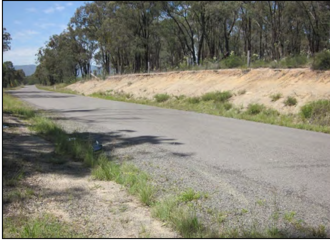
Figure 34: The cutting, looking south at MGA 319371/6380926 (IMG 1451).
