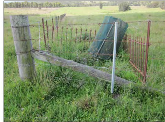
PLATE 4.30 PS15 cast iron picket fenced area, view to North
