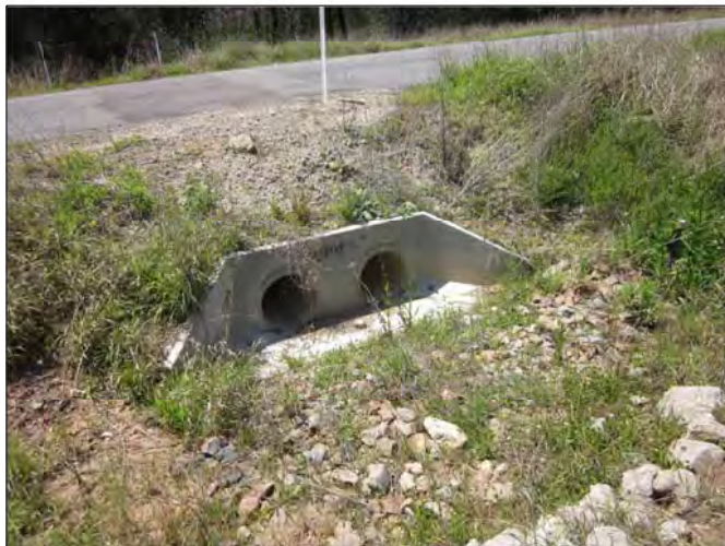
PLATE 4.43 Two-pipe culvert under Charlton Road, within realignment area, view to East
