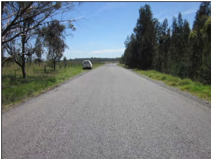
Figure 43: View north of the above culvert (IMG 1525).
