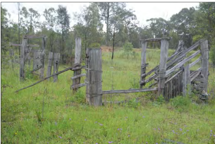
PLATE 4.27 PS12 timber yard complex, view to South-South-East
