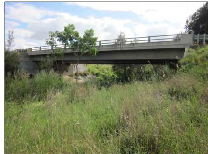
PLATE 4.40 Current bridge spanning Monkey Place Creek, view to East
