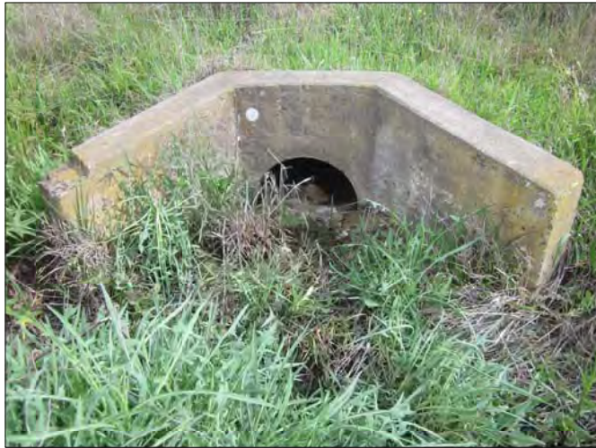
PLATE 4.57 Culvert running beneath former Broke Airstrip, view to South
