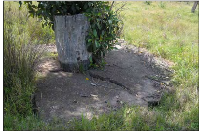
PLATE 4.10 BH16 concrete slab, view to East
