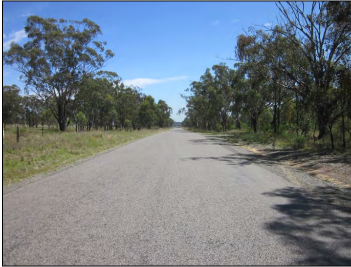
Figure 37: Looking north along Charlton Road at MGA 319092/6381365 (IMG 1473).
