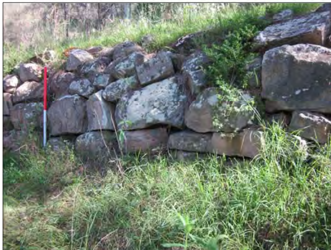
PLATE 4.67 BH13 Stone Wall alongside Monkey Place Creek, view to West (Scale = 1 metre)
