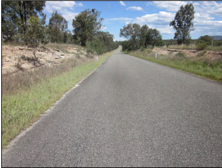
Figure 60: Looking south through the cutting at MGA 317518/6385854 (IMG 1661)
