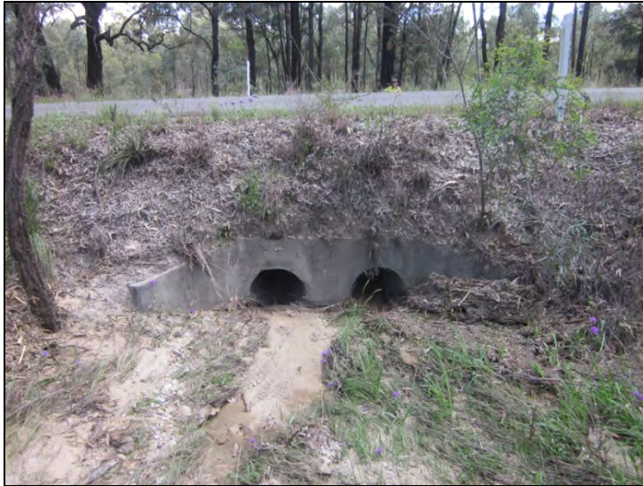
Figure 63: Culvert, western side of the road, at MGA 317279/6386539 (IMG 1678).
