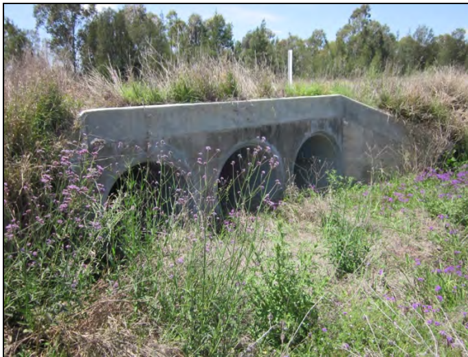
Figure 40: Three pipe concrete culvert at MGA 318758/6382269 (IMG 1504)
