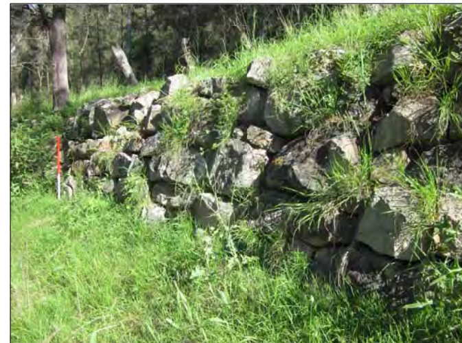
PLATE 4.68 BH13 Stone Wall alongside Monkey Place Creek, view to South (Scale = 1 metre)
