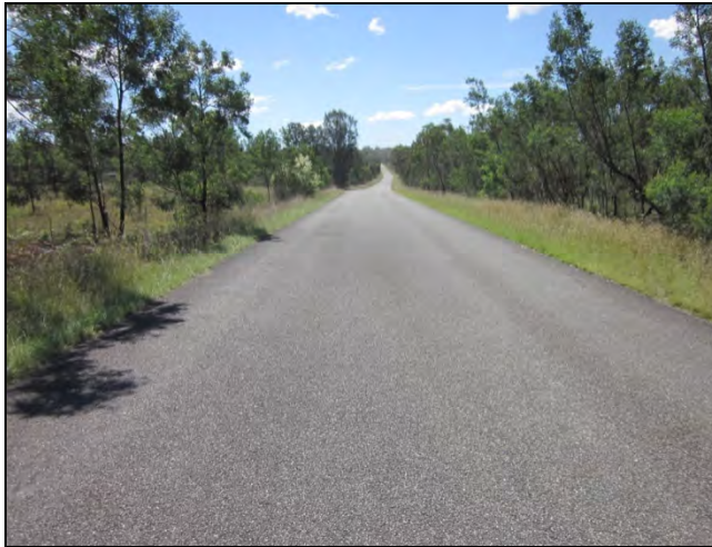
Figure 57: Looking north of the proposed realignment at MGA 317728/6385280 (IMG 1648).
