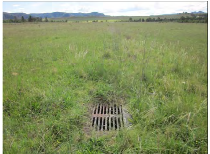
PLATE 4.55 Drain in centre of former Broke Airstrip alignment, view to West
