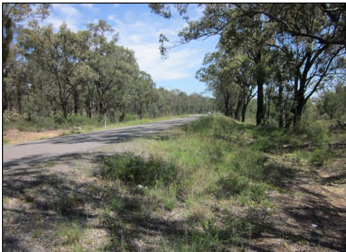
Figure 35: Fill, looking north at MGA 319327/6380989 (IMG 1457).
