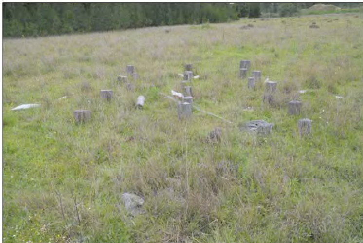
PLATE 4.15 PS4 timber footings, view to East
