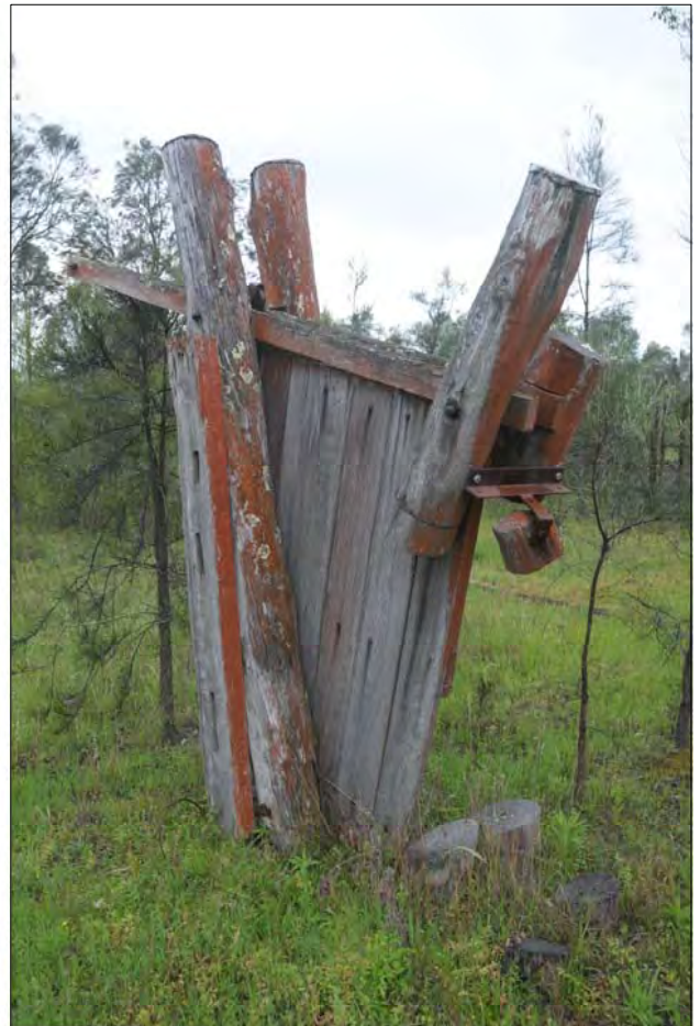
PLATE 4.28 PS12 timber yard complex, view to North-West
