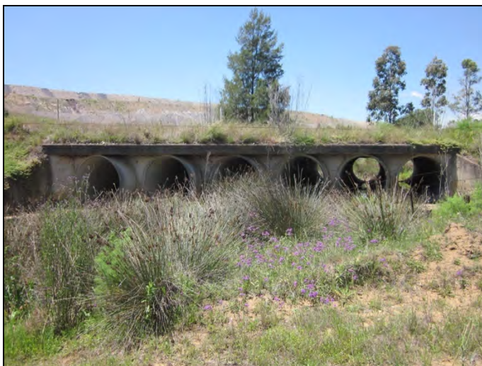
Figure 44: Six pipe culvert at MGA 318452/6383280, looking east (IMG 1544).
