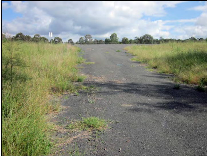
Figure 18: Looking up the original line of road to the east (IMG 1207).
