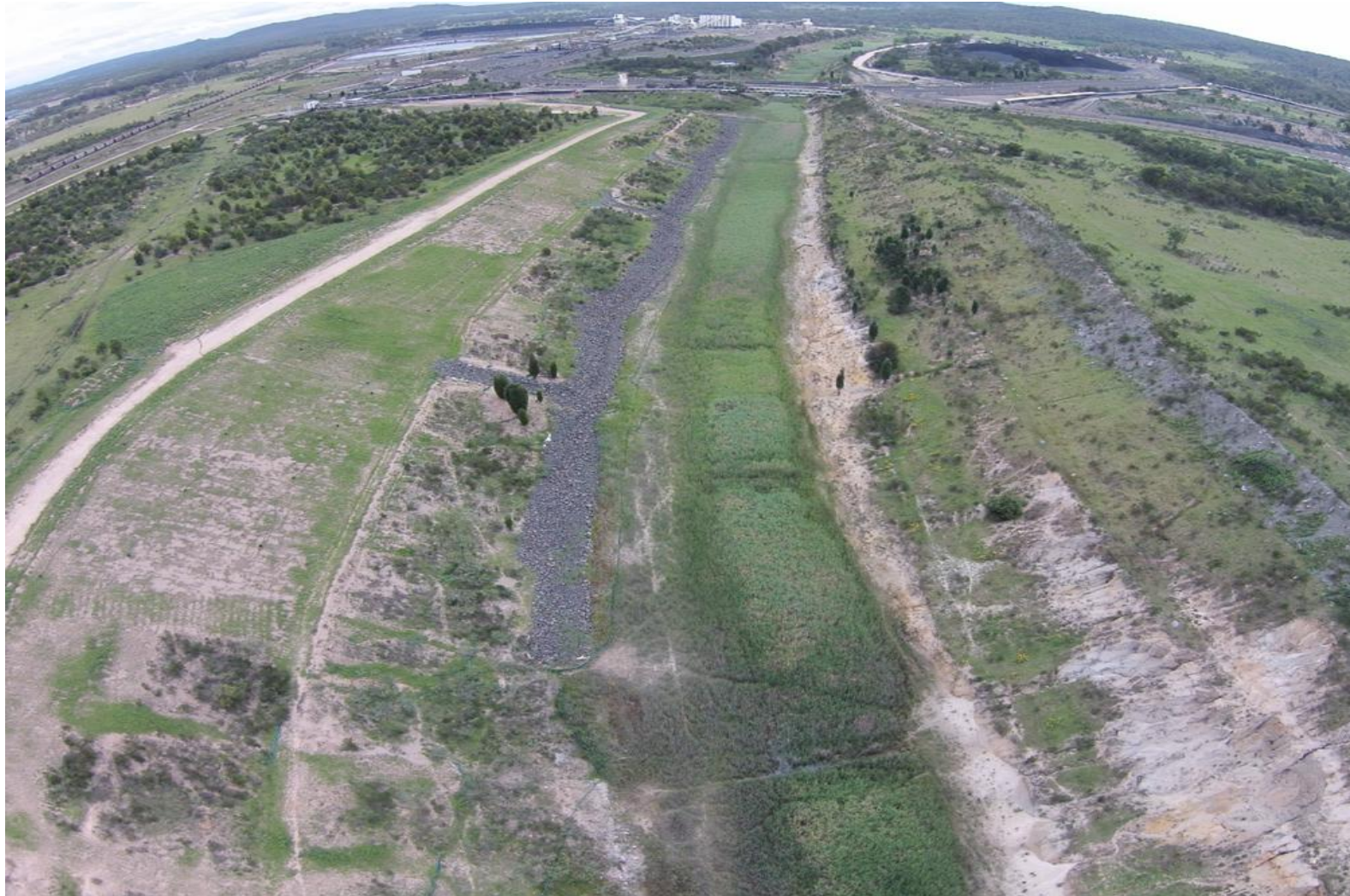
Figure 3.9 - River Remediation Pilot Area 3 Ch1000 to 1420 RHS – Completed
