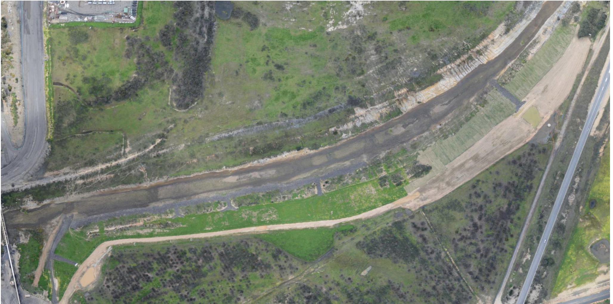
Figure 3.12– Completed River Remediation Area 3 Ch1420 to 1840 RHS
