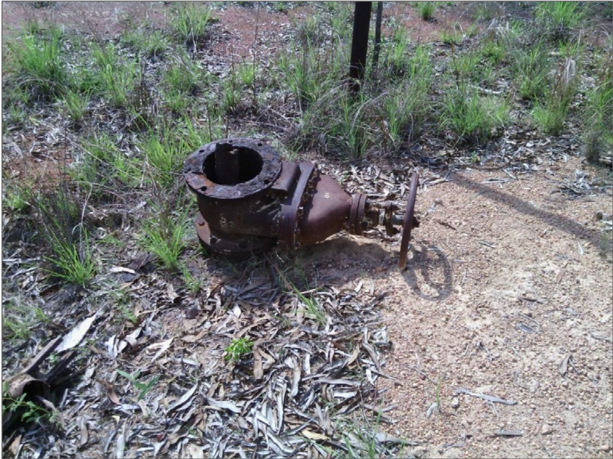
Figure A2 RN 37630 – Headworks
