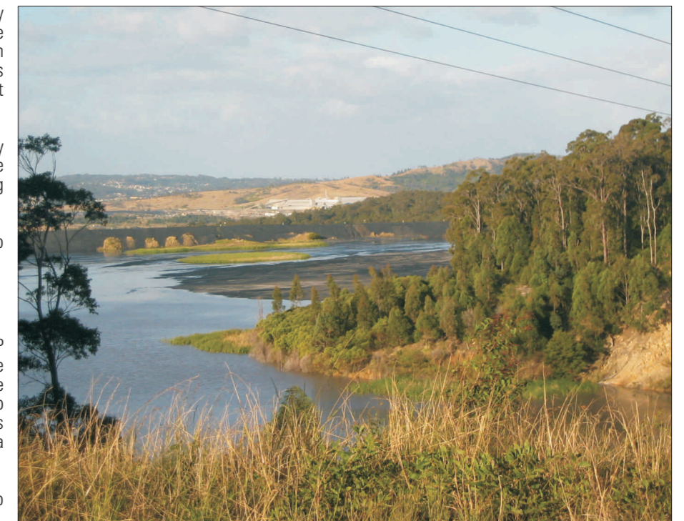
Overview of Macquarie Coal Preparation Plant Tailings Dam
